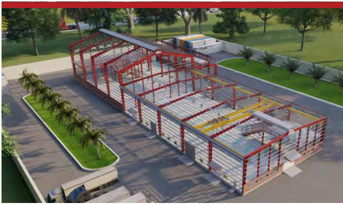
View of building without cladding
