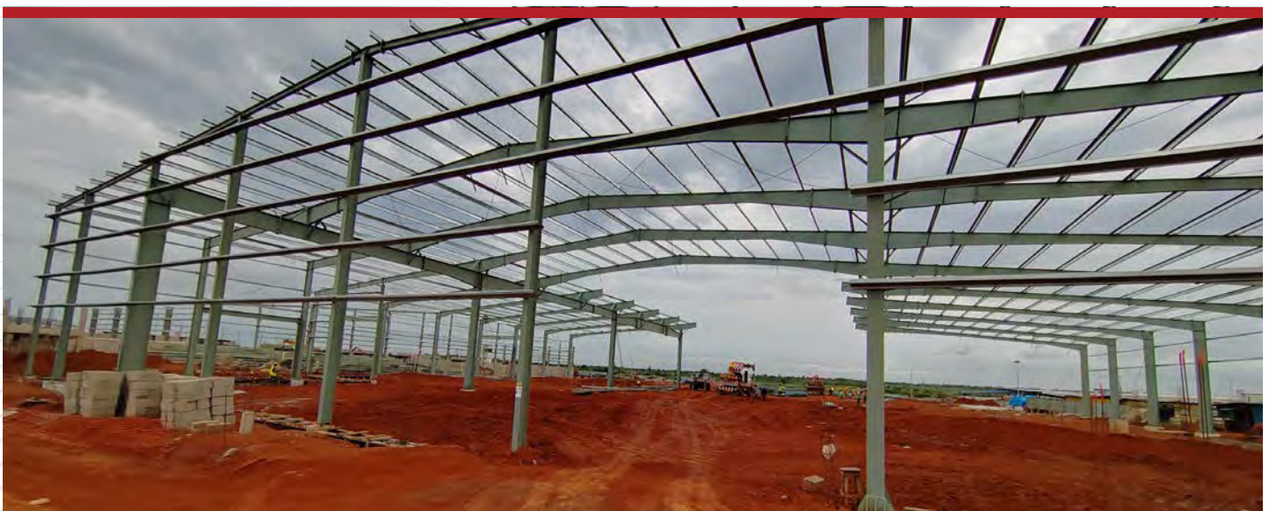
Roof installation in progress
