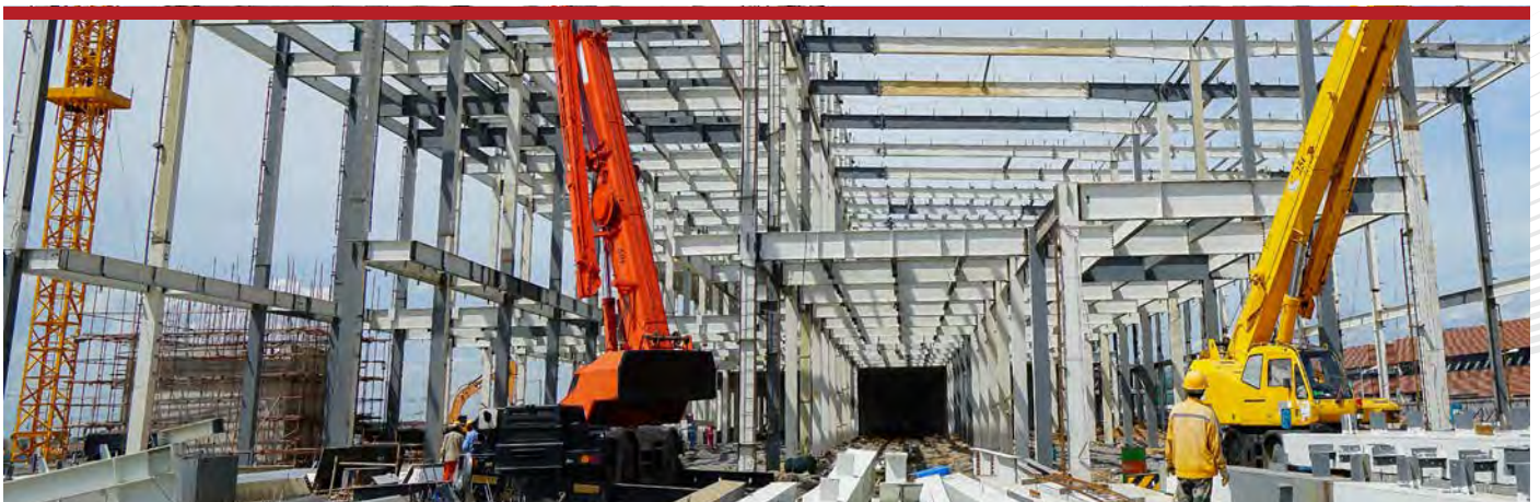
Ongoing building erection
