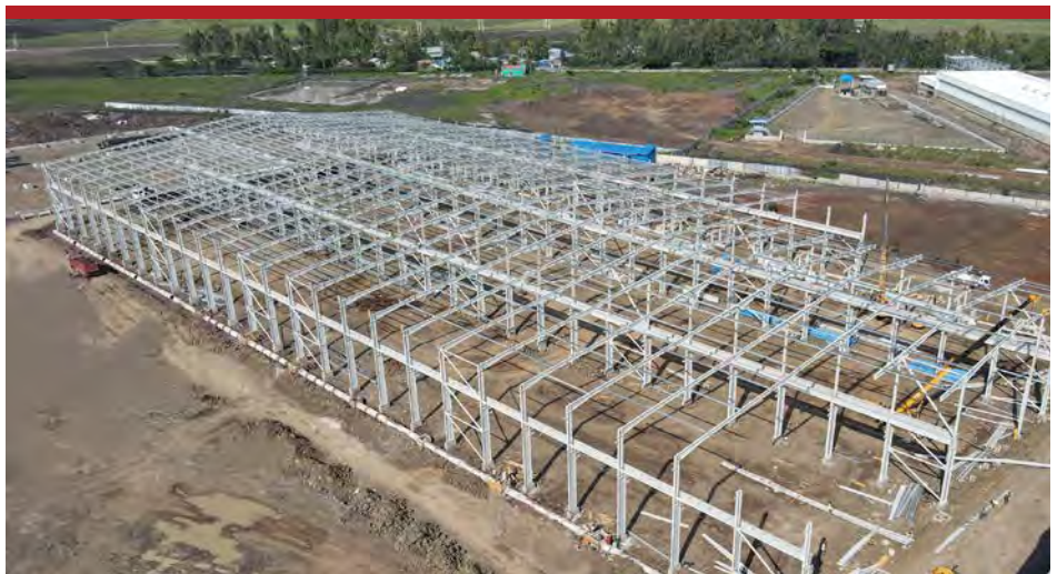
Factory warehouse assembly in progress
